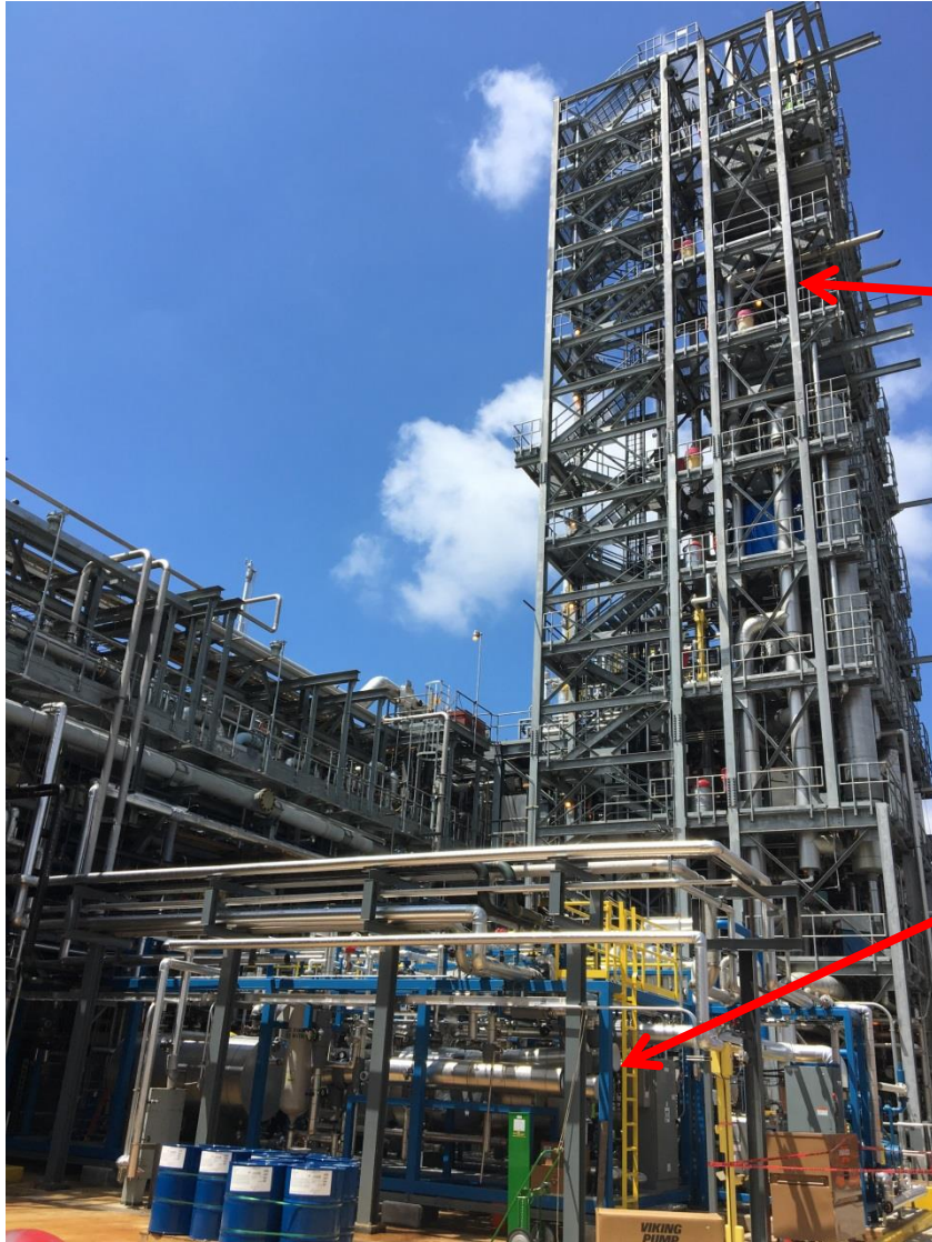
NCCC PSTU system (0.5 MW e )
